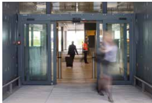
Bomb Blast Resistant Door at Heathrow Airport
